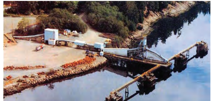
Marine load-out infrastructure
